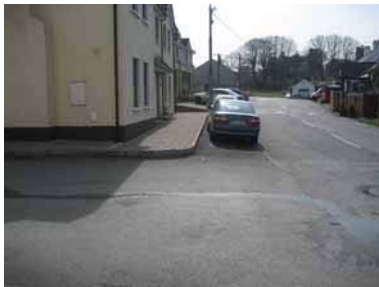
(f). Old footpath removed
