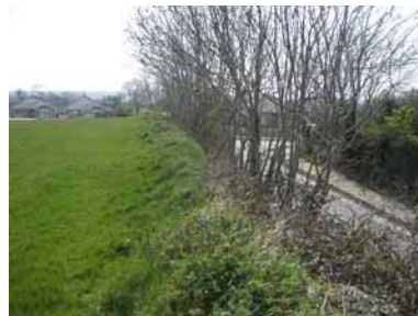
(c). Exposed fall onto road.
