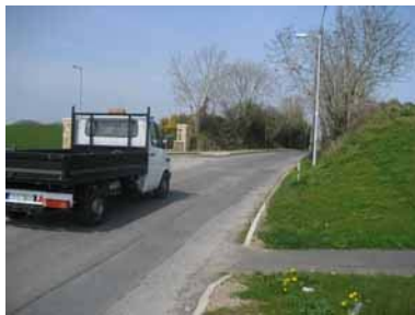
(a). Dangerous exit.
