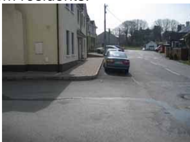
(f). Old footpath removed
